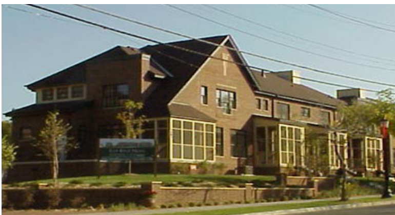
East River Mews, which includes six units of affordable housing in the Prospect Park neighborhood, was built on a former Superfund site cleaned up with state and local funding. (Minneapolis Community Planning and Economic Development)
